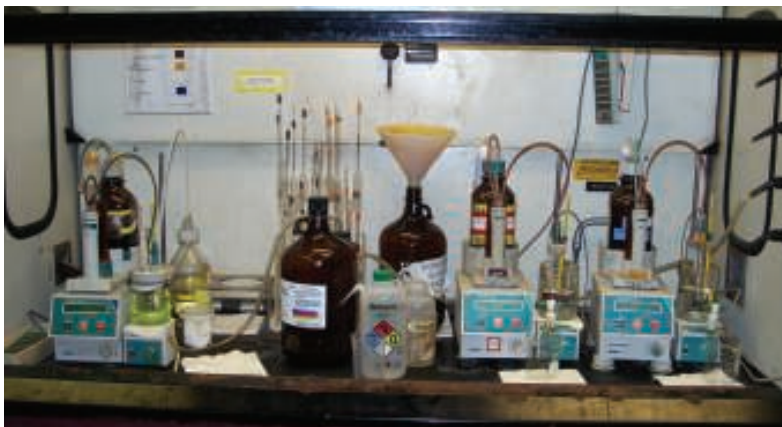
FIGURE 4. Shown here is an installation that relies on the laboratory hood for spill containment. The hazard analysis that had been carried out here was shortsighted, in that it only focused on the relatively low flowrates presented by the small volume of fluid, rather than on a potential incident that could result in an entire bottle breaking, releasing its contents
