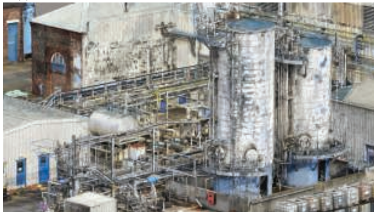
FIGURE 5. The comprehensive aerial imagery provided by a drone survey can be used to formulate a 3-D reality model of a plant
