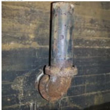
FIGURE 3. Drones can quickly provide high-resolution images for internal inspection of tanks, vessels, boilers and more
