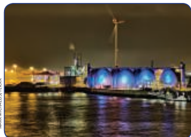
Wastewater treatment, Hamburg, Germany
