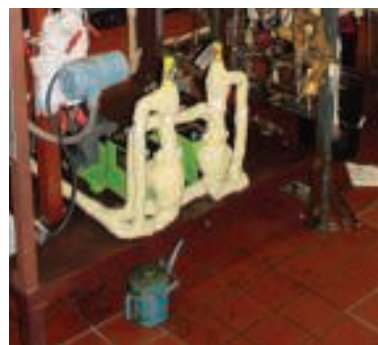
FIGURE 6. Even a well-designed pilot plant bay with floor drains will often have residual materials that could ignite near potential leaks and spill sources. If well maintained, as in this example, the residual risk should be minor
