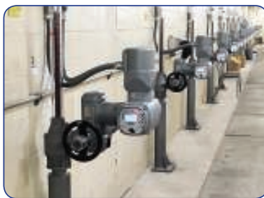
Thanks to their compact design and flexible positioning, AUMA actuators fit the narrow space between the valve stems and the wall
