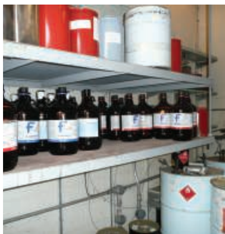
FIGURE 9. A risk assessment of this area would need to address the consequences of a smaller spill leading to a larger conflagration. While appropriately electrically classified to minimize the potential for ignition sources, the addition of a spill containment system on each shelf might significantly lower the consequences of any potential spill
