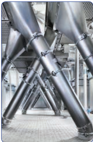
Quick-connect rings make the JACOB system easy to install and dismantle
